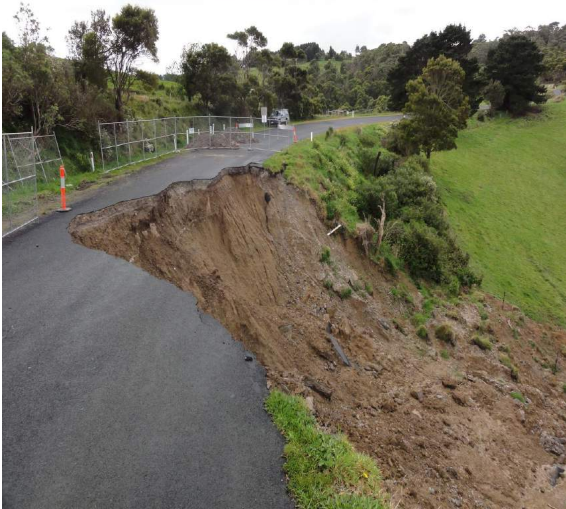
Slope Failures
