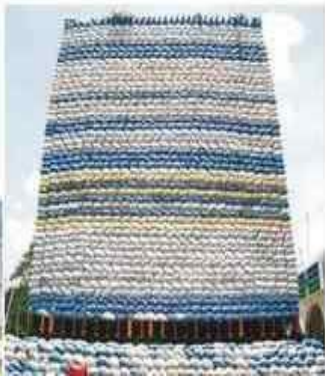
LOAD TEST BY SAND-BAGS
