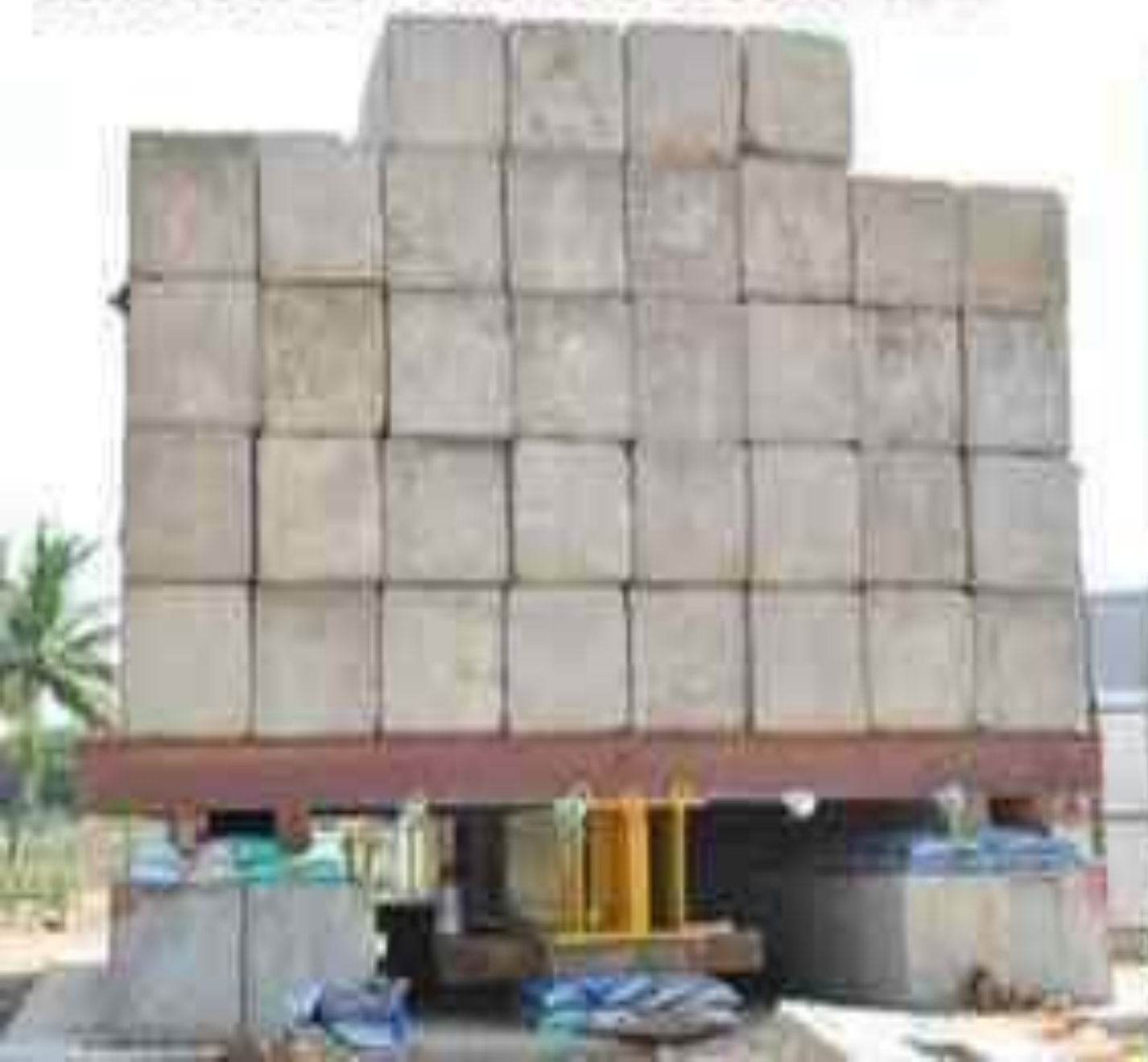
LOAD TEST BY CONCRETE BLOCKS 1000 MT
